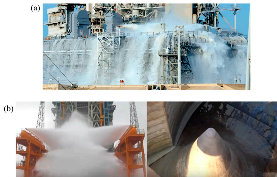
Figure 1. Schematic diagrams of water spray systems for launch sites: (a) the Kennedy Space Center; (b) the Wenchang Spacecraft Launch Site.
