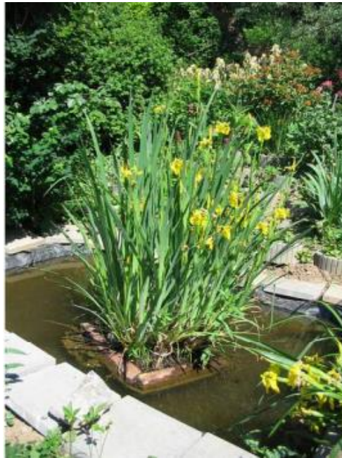
Fig. 3. Small natural wastewater treatment plant without outflow (final treating tank with floating islands with yellow hyacinth) forms an aesthetic element in the garden [46]
