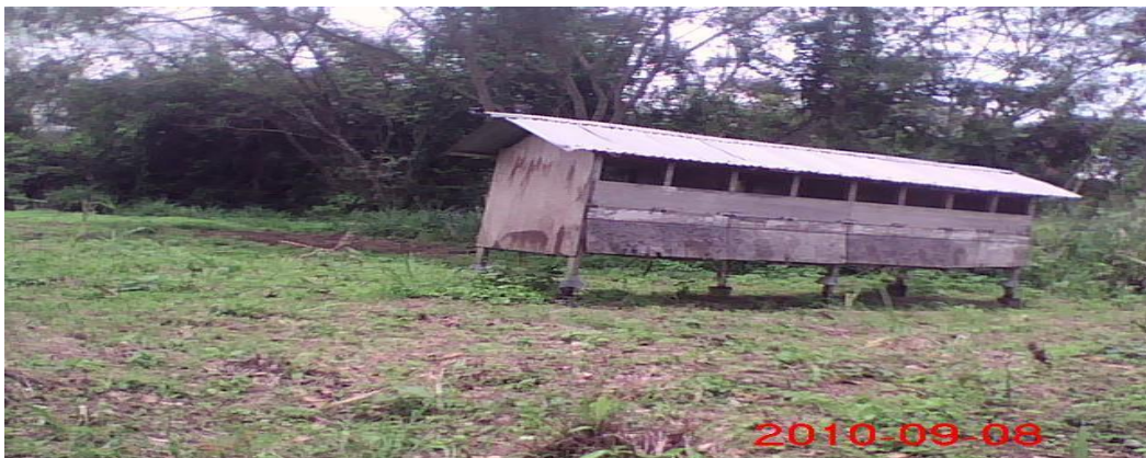
Fig. 1. Back view of the 45° orientation building with eight pens showing leeward 20% opening ventilation
