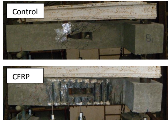
Fig. 10. The effect of FRP strengthening on the cracking distribution of tested RC beams
