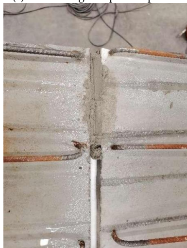
(e) Smoothing out the mortar
