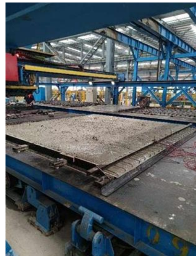
(b) Pouring concrete to form a precast plank
