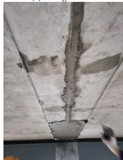
(f) Applying a layer of mortar
