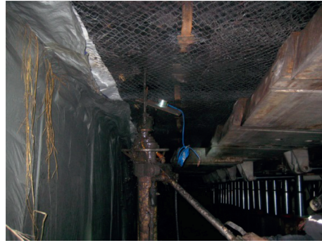
FIGURE 15: Installation of the roof pressure sensor.
