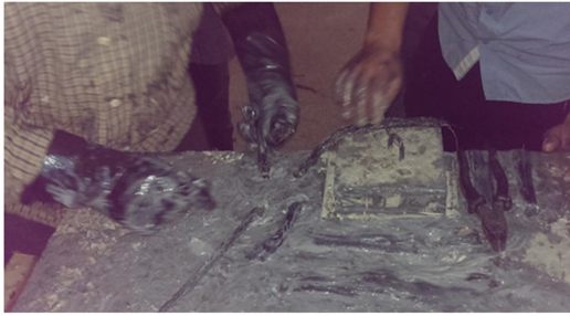
Fig. 4. Manufacturing of GFRP stirrups
