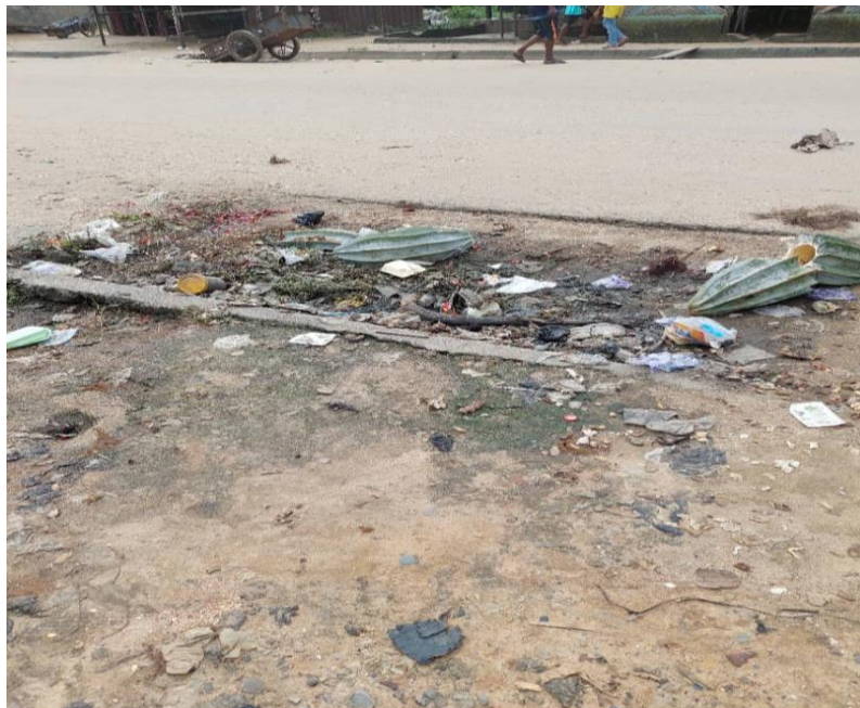
Plate 1. Debris filled drainage in Umuechem community causing flooding on the adjoining farmlands
